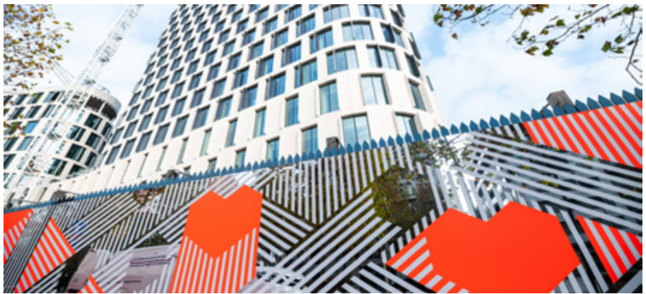
Art Of Love - Quatuor building site - Brussels North area
